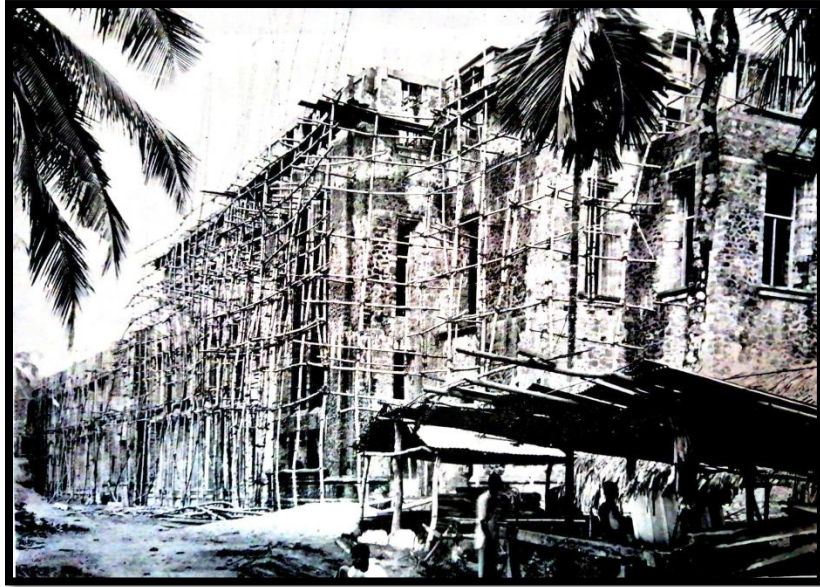
Construction of main block
